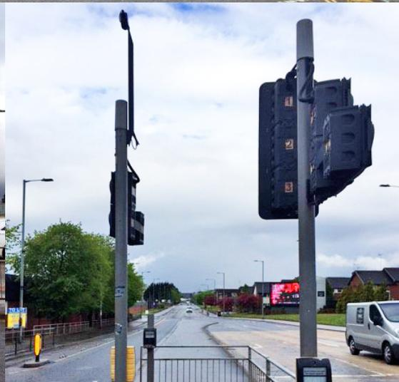
The council's contractor mounted a TMB-134 detector at the top of an existing traffic signal pole at the intersection. The engineers were then able to set up the device using the existing cabling, defining up to 9 virtual zones to detect vehicles approaching the intersection. These zones could be set to detect on individual lanes, including right or turn left lanes.
